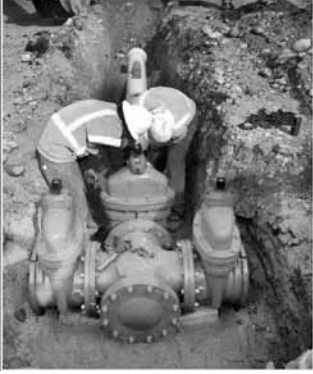
Installation of purple pipe
