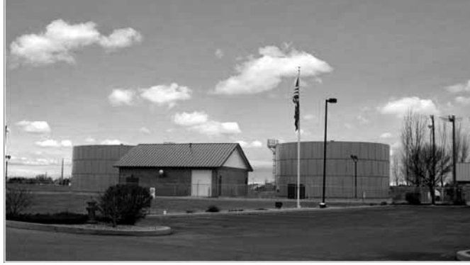
Meridian reclaimed water booster station
