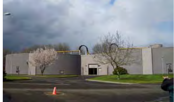
COLUMBIA BOULEVARD ANAEROBIC DIGESTERS
